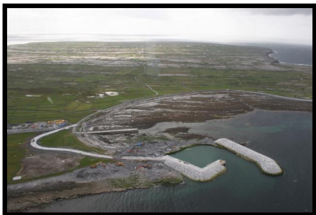
Development of the Harbour at Caladh Mór, Inis Meáin
